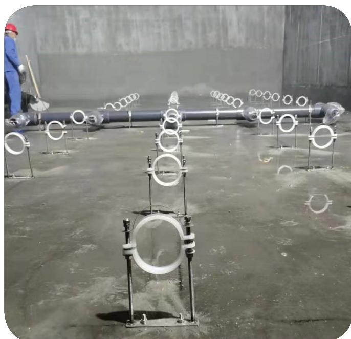
Pic. 1. During installation
